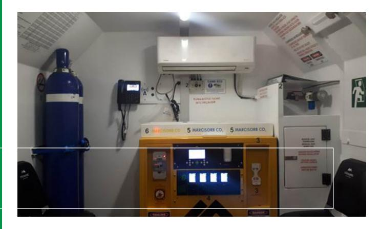
Pictured: Aura-FX DGM and Series IV Scrubber inside the mining refuge chamber.
